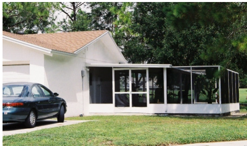
Unacceptable: prefabricated screen room.
