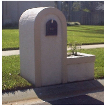
Unacceptable: Large stucco, brick and/or stone mailbox structure
