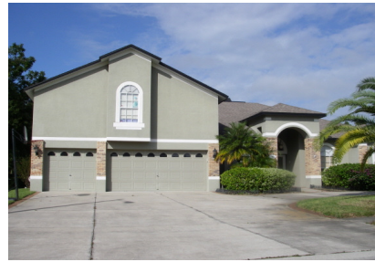
Unacceptable: "lopsided" upper floor on one side
