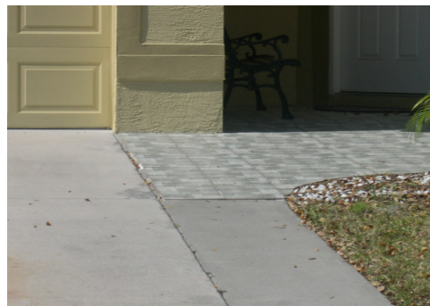
Acceptable: entryway and extension are different applications however driveway extension is concrete
