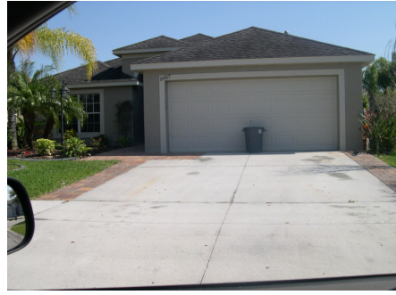
Unacceptable paving extending into driveway
